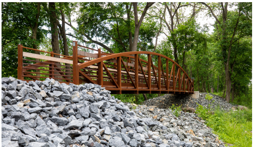
Contech Capstone style pedestrian bridge
